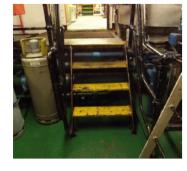
On these stairs, a person reached the bottom step, and his left foot slipped from the tread, landing heavily on the deck injuring his foot
